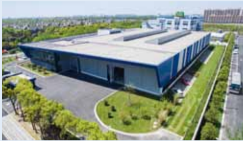
The new factory site of Aerzen Int. Trading
