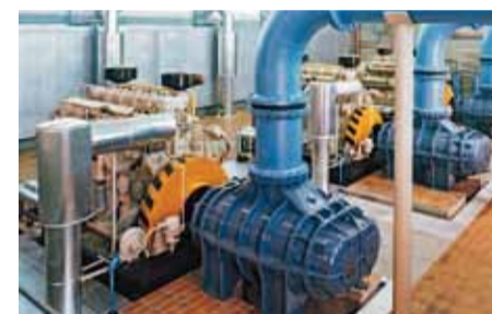
In the environmental engineering field AERZEN began to supply components, e.g. positive displacement blowers type GMa 18.17 for the aeration of sewage basins.
