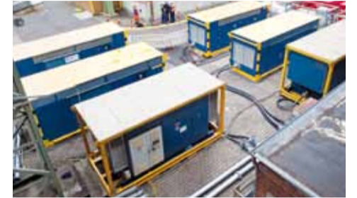
Rental unit from AERZEN International Rental with six oil-free compressing AERZEN screw compressors for preliminary conveying air supply
