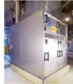
Conveying air station of Zellstoff Stendal GmbH with the rotary lobe compressor of the new series Delta Hybrid Generation 5 supplied by AERZEN
