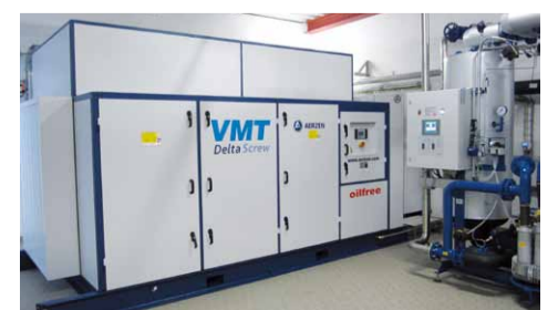
For the food industry: a VMT 1 L compressed-air assembly with compressed-air drier and compressed-air filter
