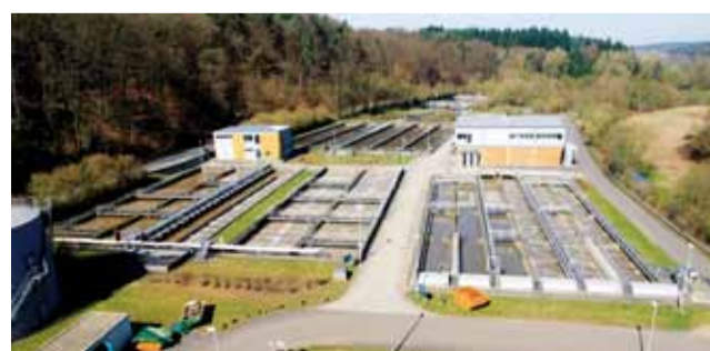
View onto the three activated aeration basins
