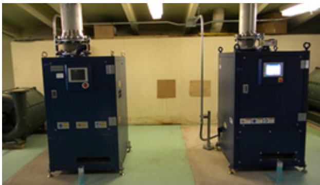
Dmuchawy Aerzen Turbo TB100 w oczyszczalni "Blue River" w Silverthorne, Colorado
